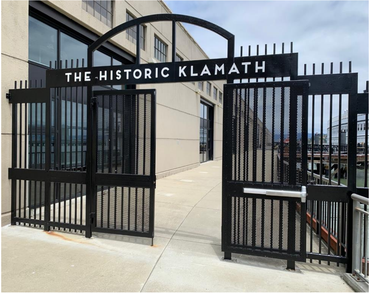
Figure 3: Pier 9 public access area from gate at the Embarcadero.
