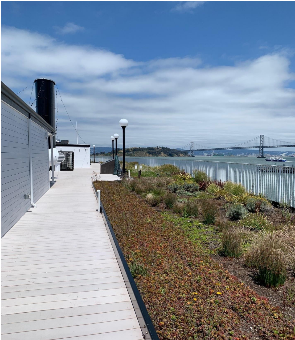
Figure 6: roof deck public access area
