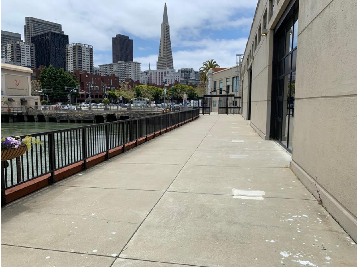
Figure 5: Pier 9 public access area from near gangway
